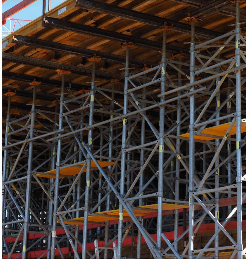
Formwork in concrete construction is used as a mould for a structure in which fresh concrete is poured only to harden subsequently. Types of formwork for concrete construction depends on formwork material and type of structural element.
